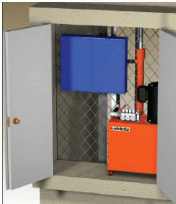
Figure 4: Power unit placed in wall closet allowing natural oil cooling with every elevator car movement (courtesy: Leistriz)
